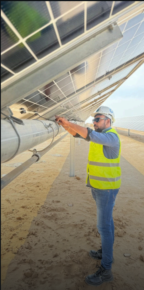
Wiring & commissioning support
