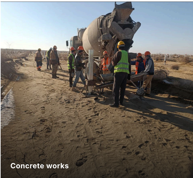
Structural mounting and civil works in progress
