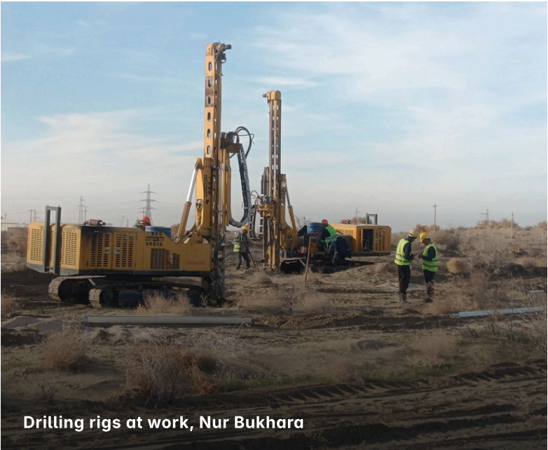
DTH drilling rig
